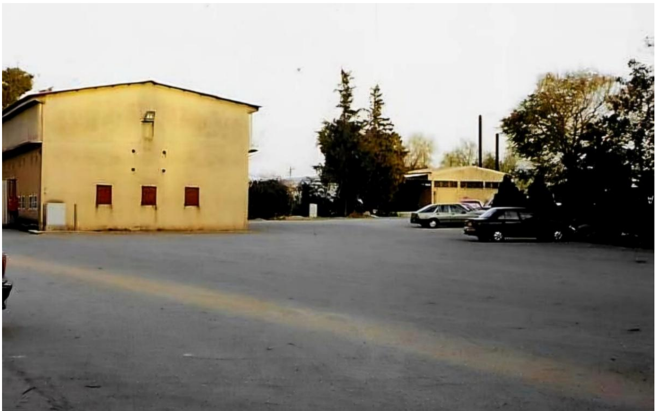
Sports hall (old Granary), parking lot, and steam room from 1984.
